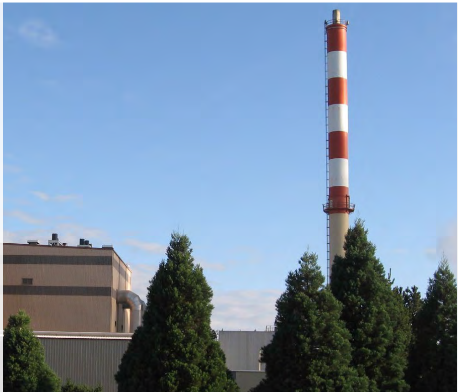
The Marion County WTE facility has provided reliable power since 1987. Photo courtesy of Marion County
