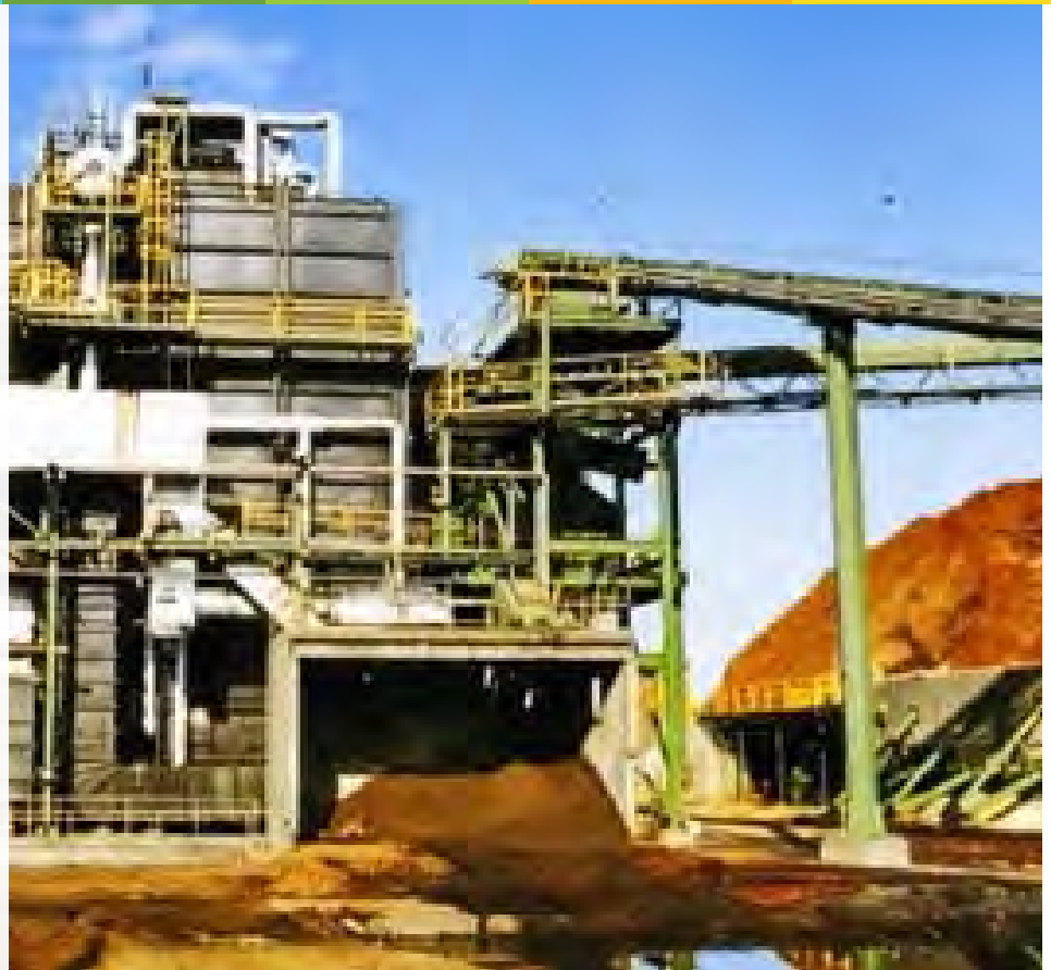
Biomass One turns 355,000 tons of wood waste into 30 MW of electricity. Photo courtesy of Biomass One
