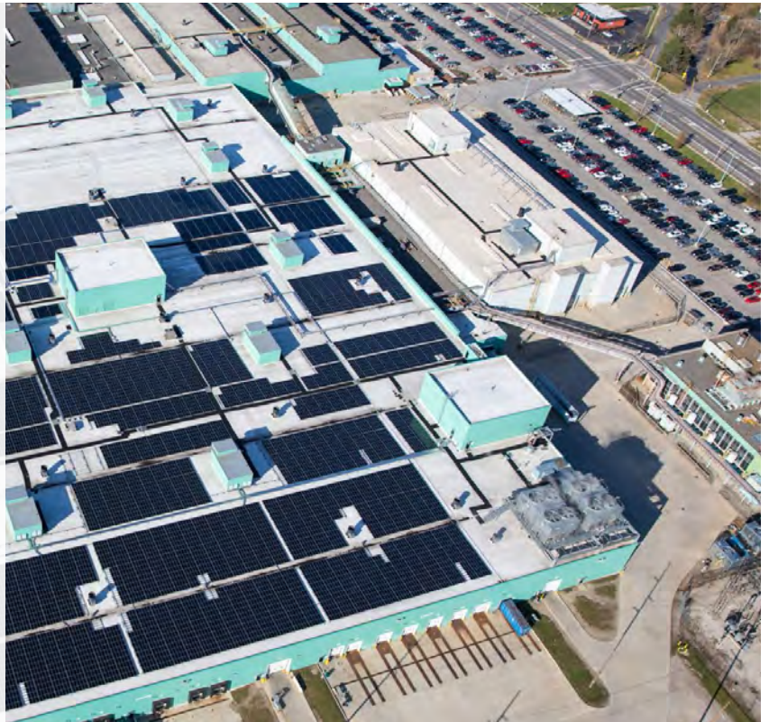
The General Motors Toledo Transmission plant will save $40,000 annually as a result of its investment in a 1.8 MW rooftop solar array. Photo courtesy of General Motors.
