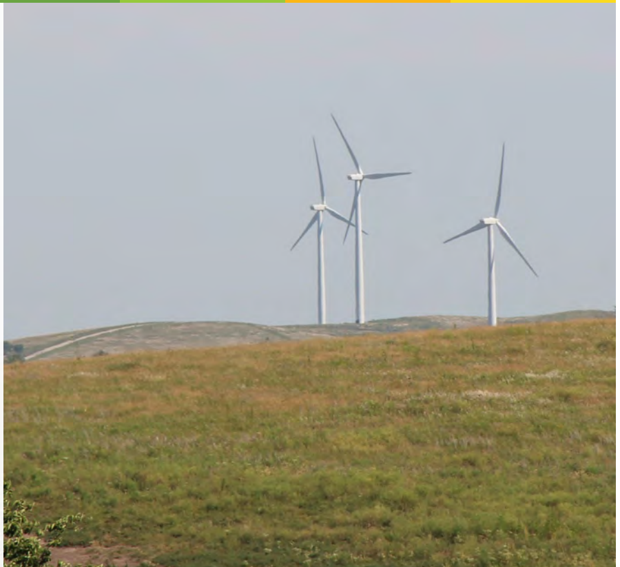
The Broken Bow wind farms generate enough renewable electricity to power 55,000 homes. Photo courtesy of Midwest Wind Energy.
